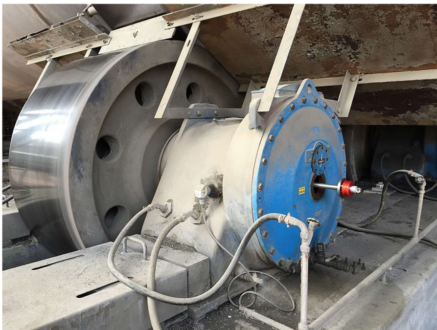
Fig.10.1.2 Ball prism attached to the roller shaft
