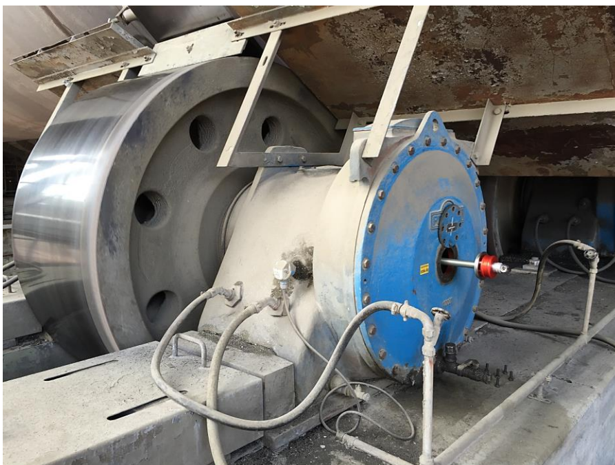
Fig.10.1.2 Ball prism attached to the roller shaft
