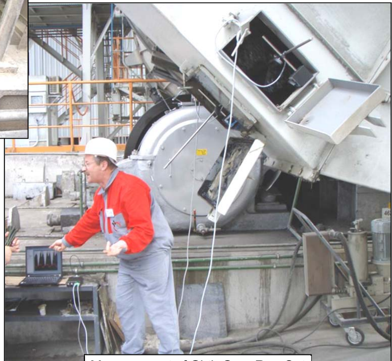
Measurement of Girth Gear Run-Out
