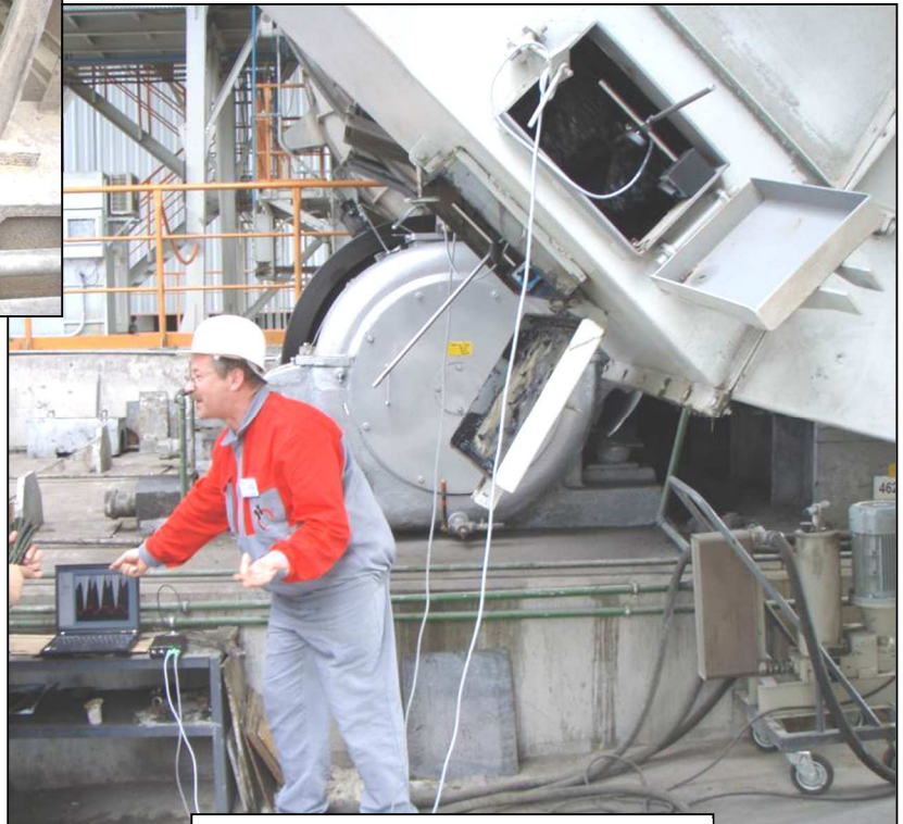
Measurement of Girth Gear Run-Out
